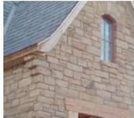
Cornice Return – Acceptable
